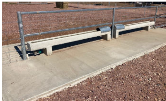
FIGURE 24: Croc trough pump set up to reticulate water around the trough and reduce dust film. (Source: croctroughpumps.com.au).
