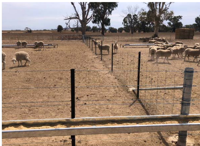
FIGURE 3: Steel posts and ringlock fencing with plain wires where stock need to access the trough in the fenceline.
